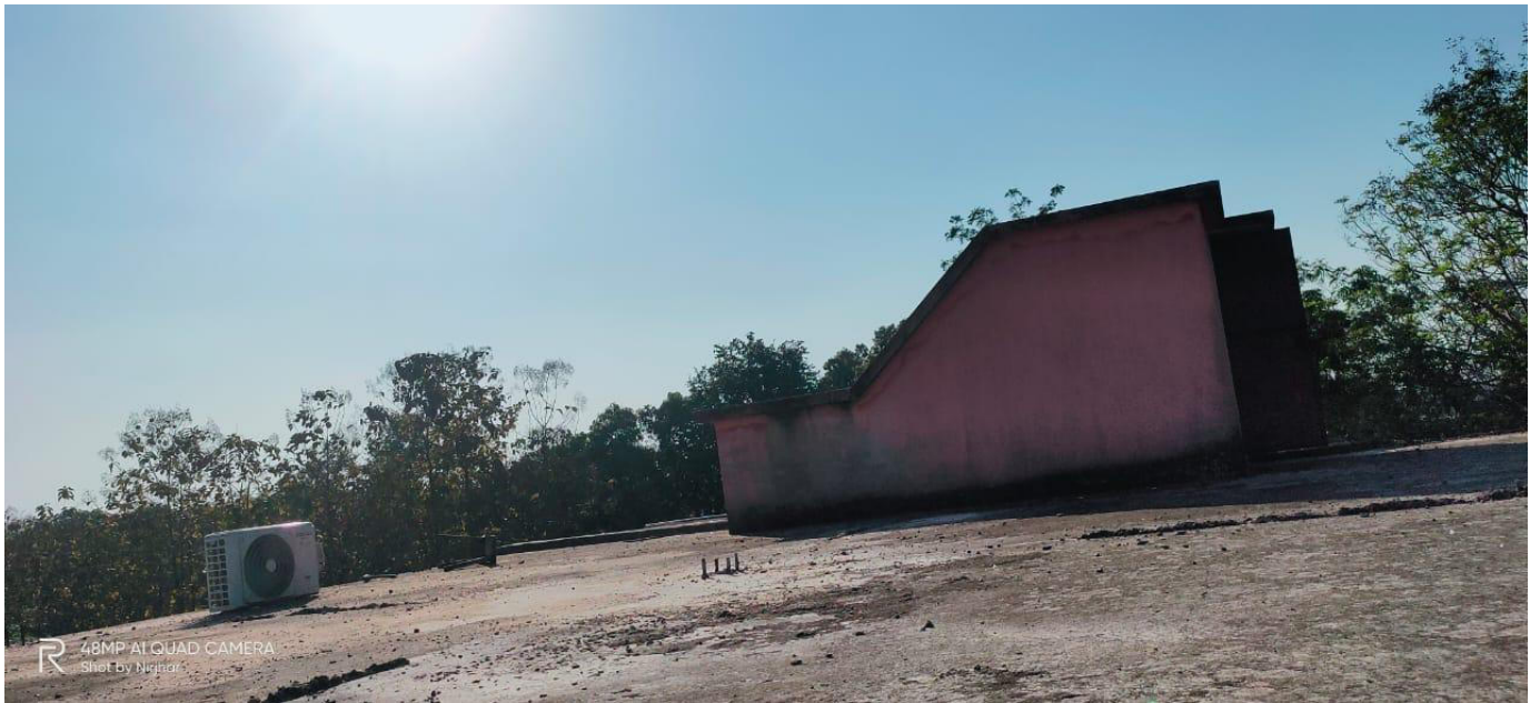
(Proposed Site for installation of rooftop solar Power Plant)
