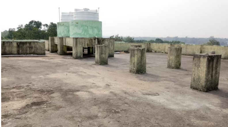
Space for solar Rooftop Plant in block-2.
